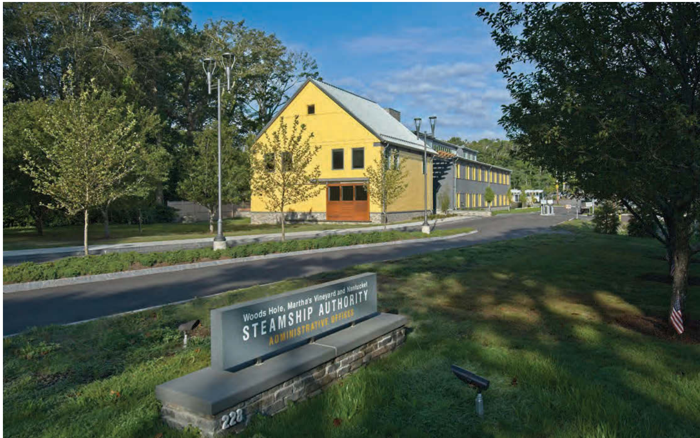
New SSA Administrative Office Building (2018)
