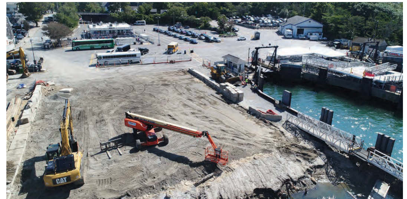
Slip Reconstruction - Phases 2-4 (2018-2021)
